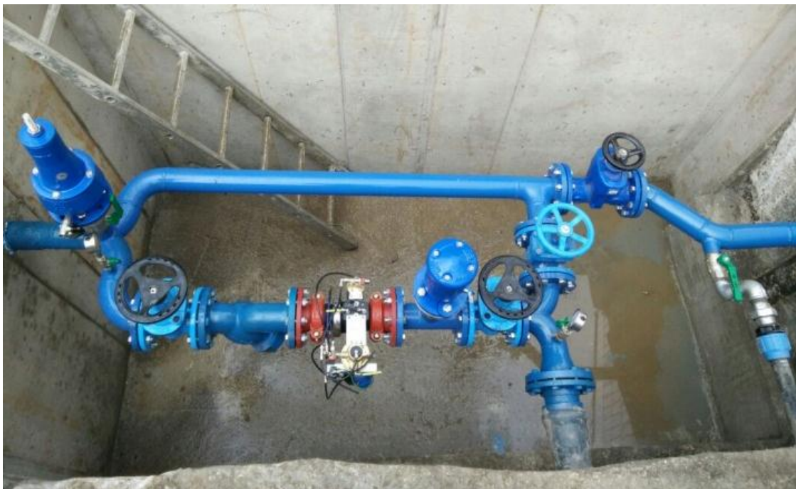
Figure 7 – Typical installation of a PRV.
